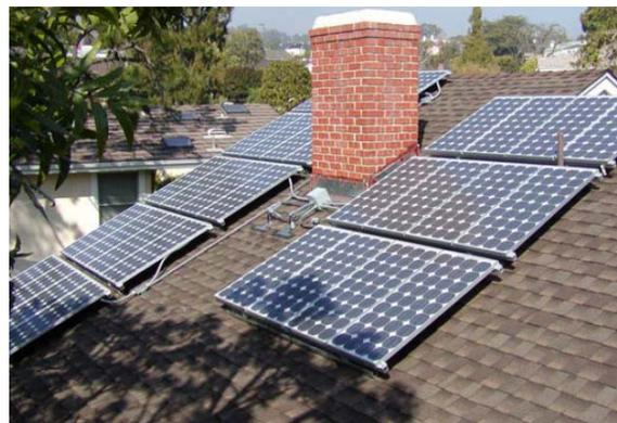
Figure 1.4: Shadowing of PV Cells [14]
